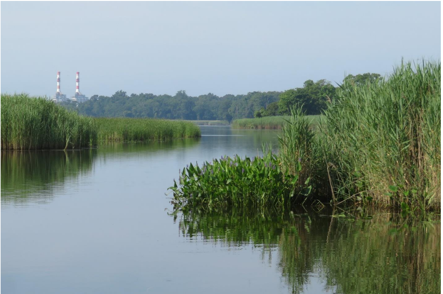
Figure 8: View from a tributary of Dundee Creek with the Charles P. Crane Generating Station behind
