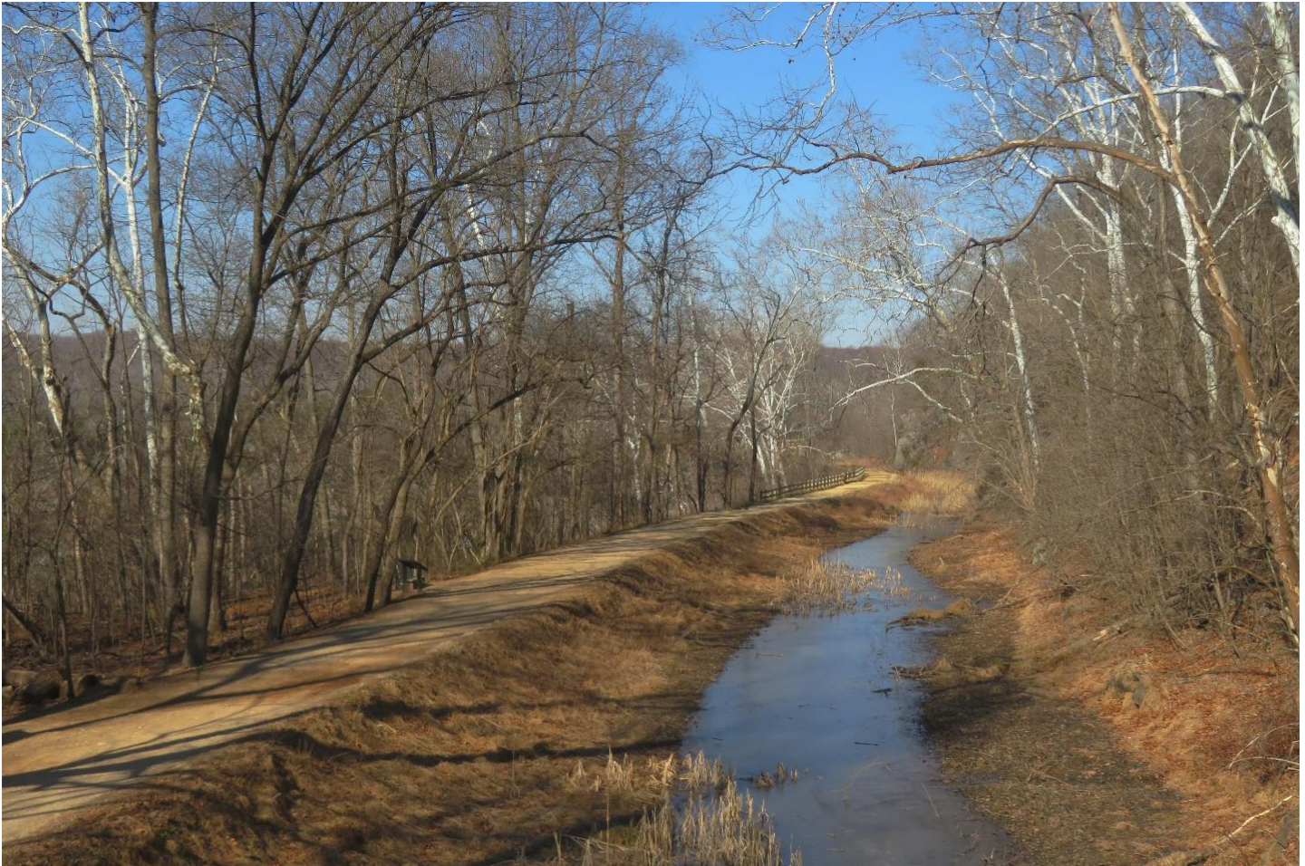
Figure 10: C&O Canal and towpath
