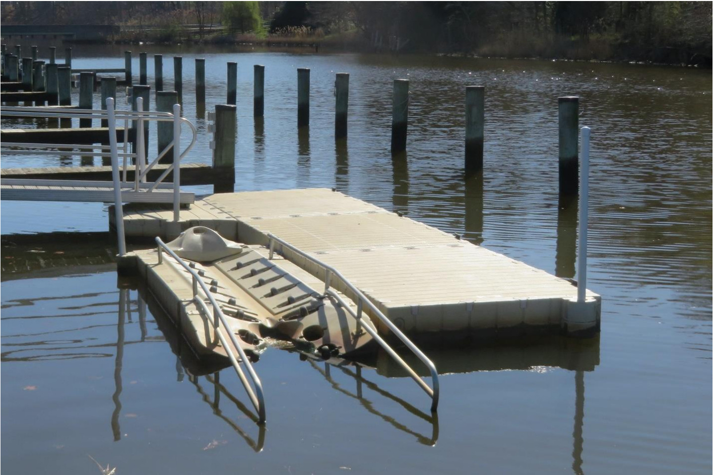
Figure 2: Centreville Wharf floating dock
