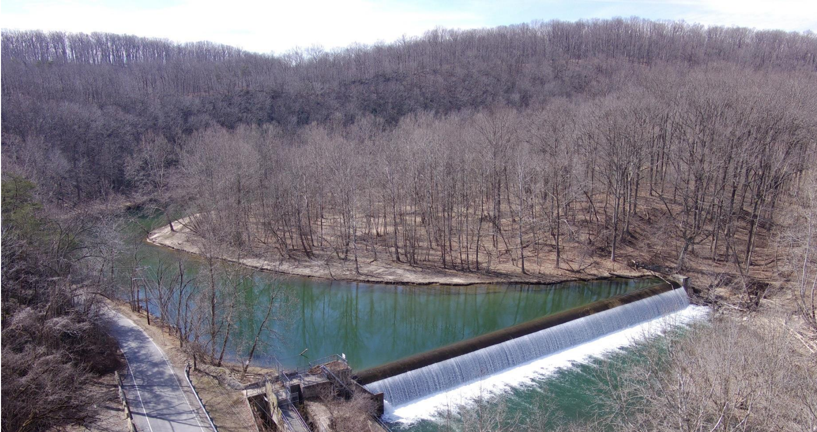
Figure 1: Daniels Dam on the Patapsco River
