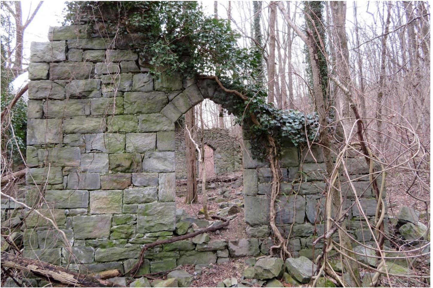
Figure 5: Stone ruins of the Saint Stanislaus Kostka Catholic Church
