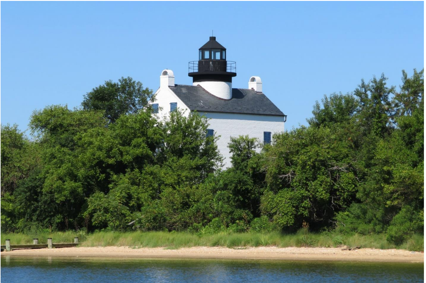
Figure 3: Blackistone Island Lighthouse replica
