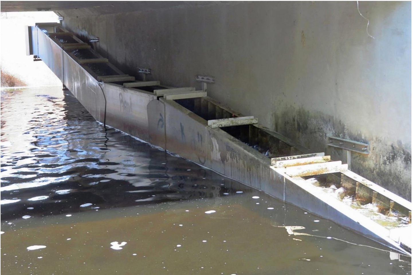
Figure 9: Fish ladder under Galestown-Reliance Road
