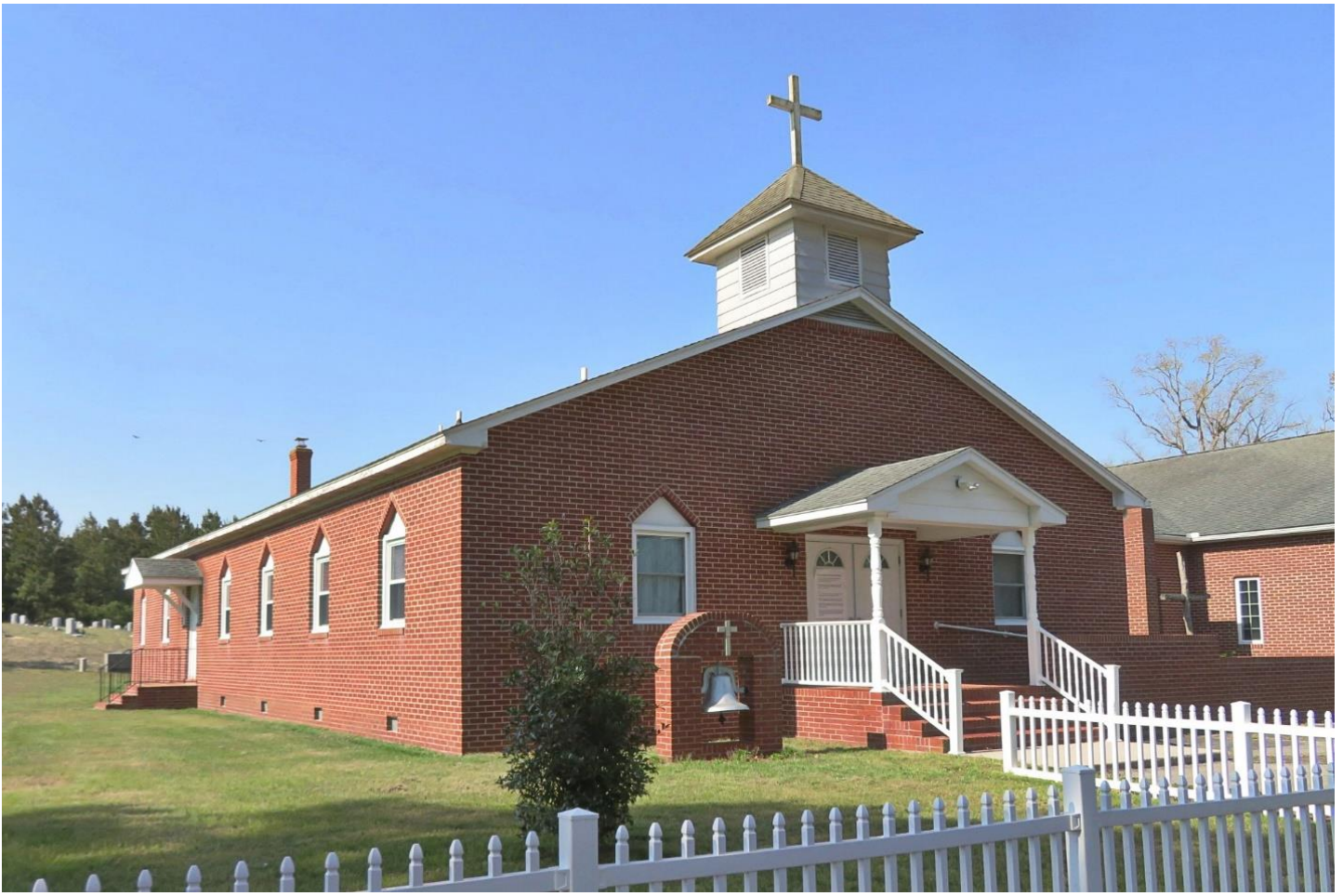
Figure 11: Zion United Methodist Church in San Domingo
