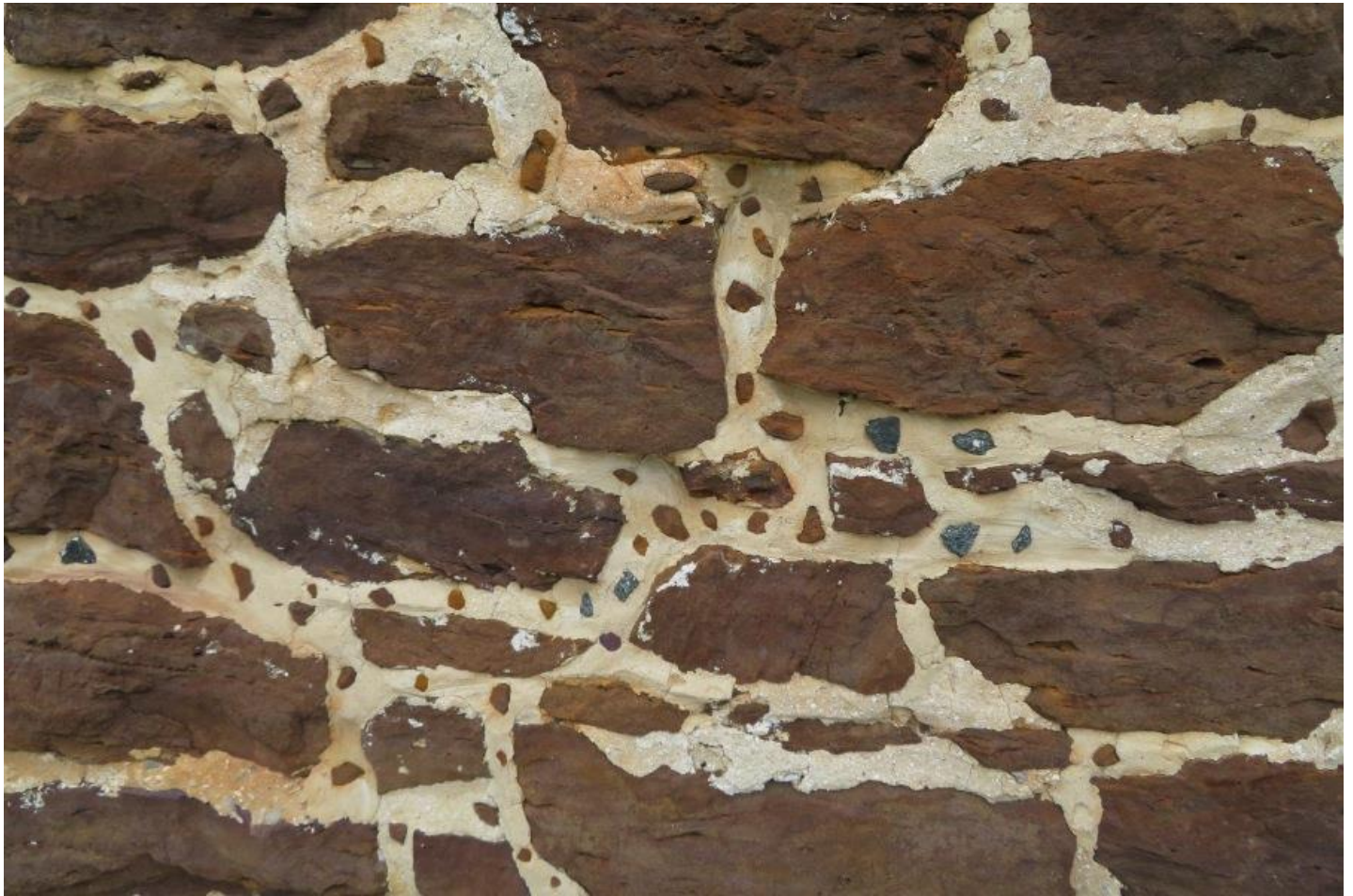
Figure 4: Galleting in the stone farmhouse
