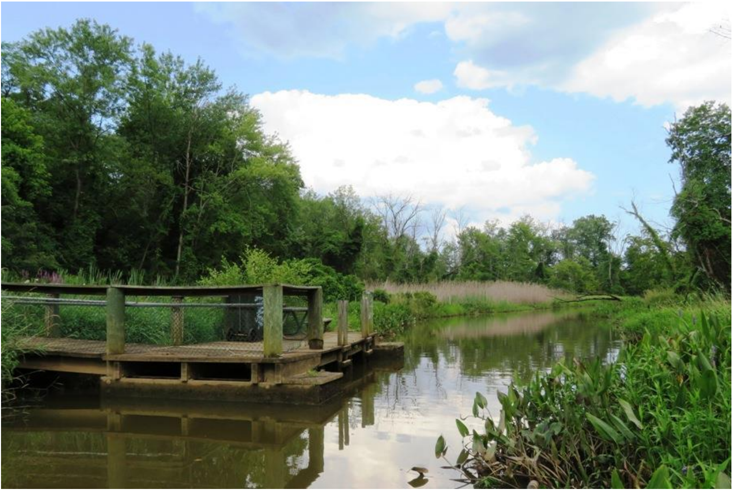
Figure 5: Colman Manor pier on Dueling Creek
