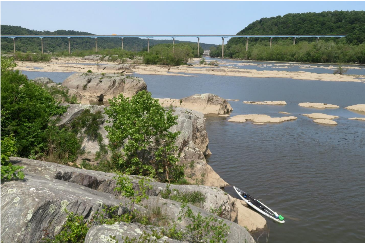
Figure 13: Norman Wood Bridge (Route 372) in the background
