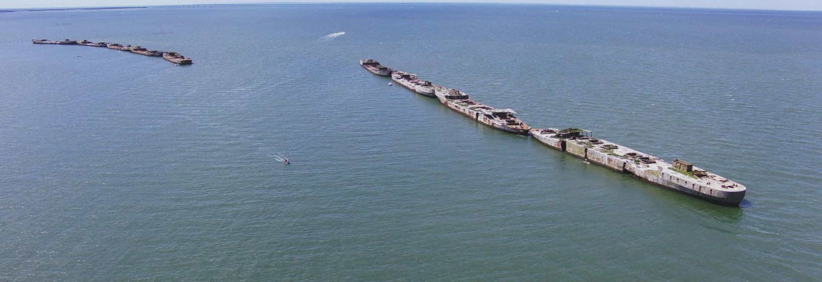
Figure 1: Breakwaters created by sunken concrete ships
