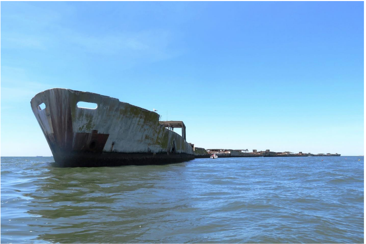
Figure 4: The S.S. Willard A. Pollard at the end of a chain of concrete ships forming a breakwater
