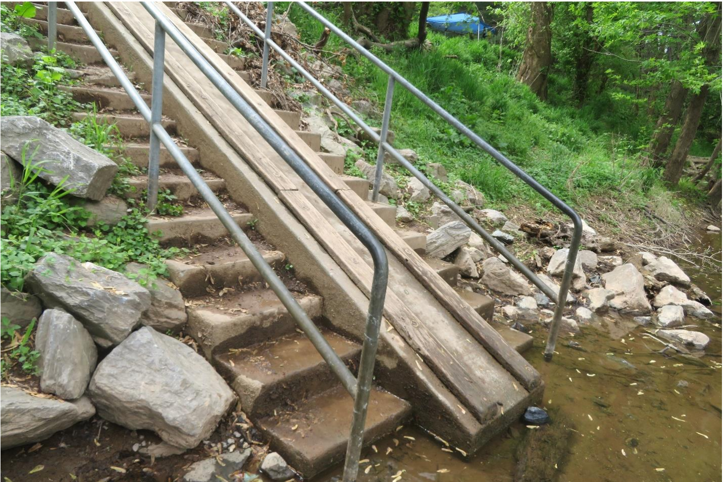
Figure 2: Non-vehicular ramp with staircases at Buckeystown Community Park
