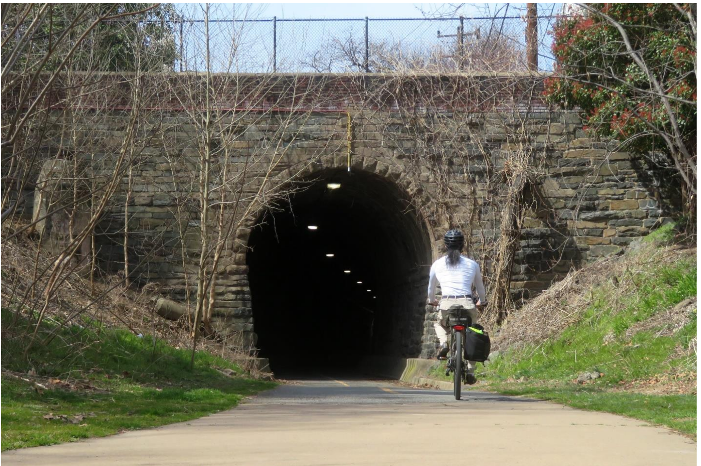
Figure 4: Wilkes Street Tunnel in Old Town Alexandria
