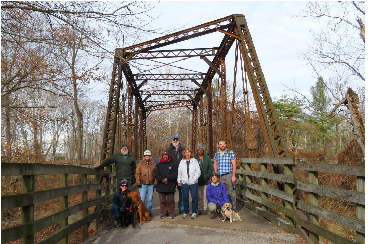
Figure 4: Pratt Through Truss Bridge
