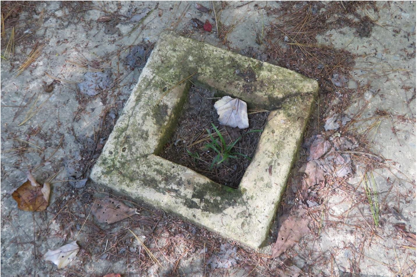
Figure 8: Concrete structure remnant from amusement park
