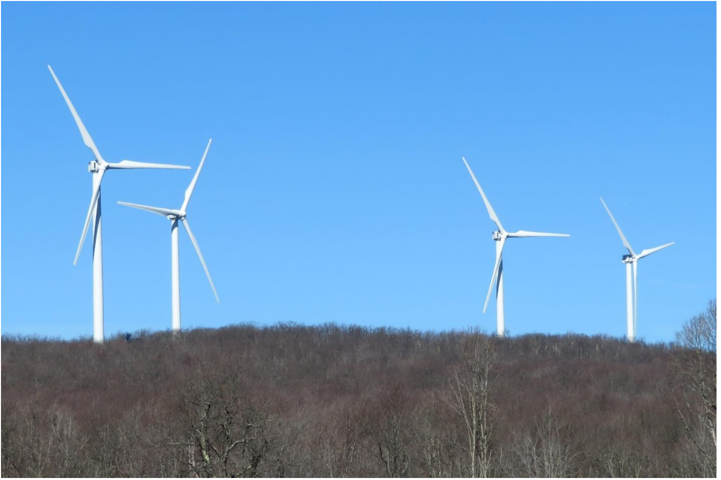
Figure 5: Wind turbines on Backbone Mountain
