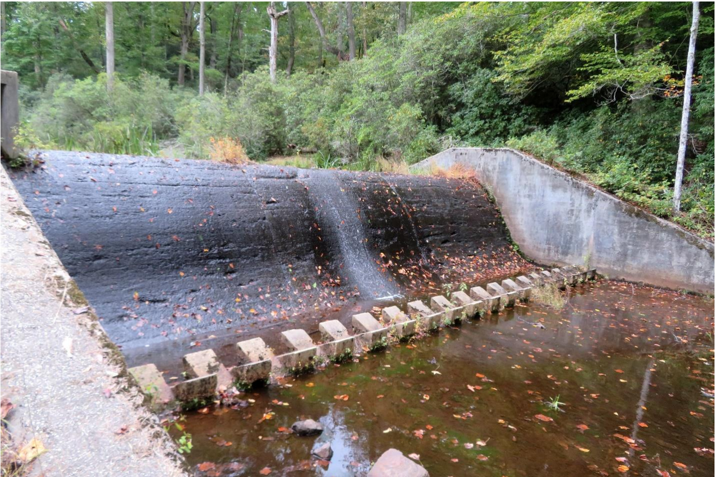
Figure 6: Overflow dam at Rock Spring Pond
