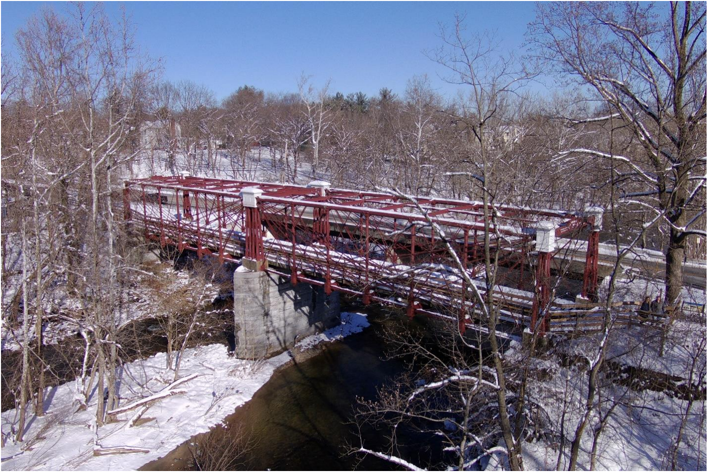
Figure 9: Winter view of the last surviving Bollman Truss Bridge
